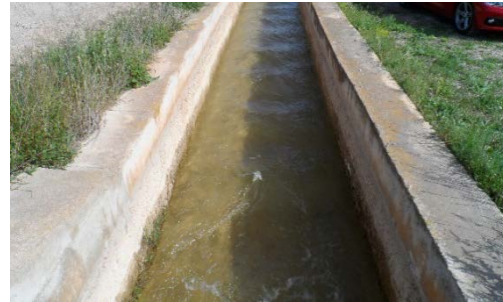
Fig. 4: Supercritical flow channel, v = 5.5 m/s
