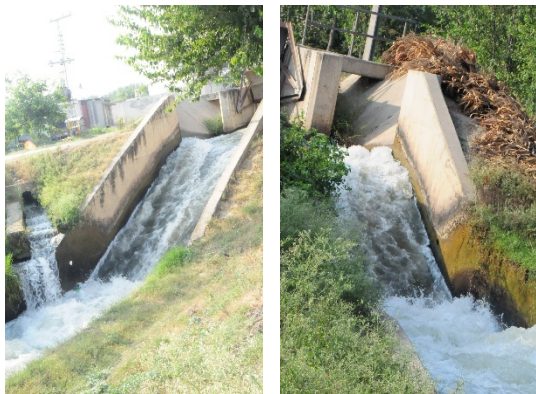
Fig. 5: Two typical drop structures (pictures courtesy of A Anwar, IWMI Lahore)
