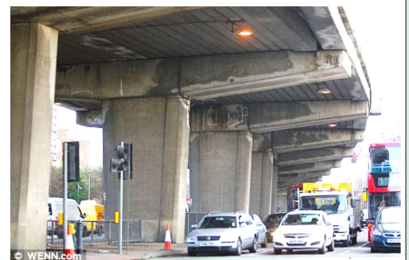
Rebar corrosion - A4 elevated section, London, UK.
