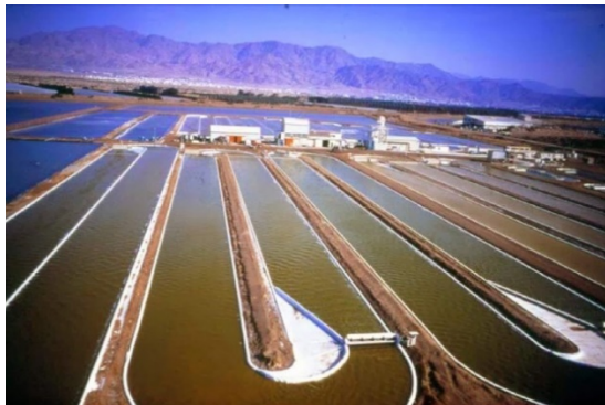
Fig. 1: Typical raceway type algae pond
