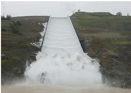
Fig. 1: Oroville dam spillway
