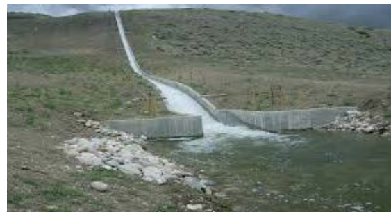
Fig. 2: Steep chute in an irrigation canal in Wyoming
