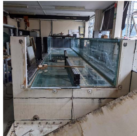
Fig. 3: Removal of old wave tank
