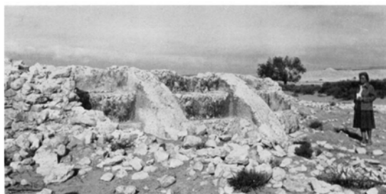
Fig. 3: Soil retention dam with buttresses (Taregat basin, Tripolitania)
