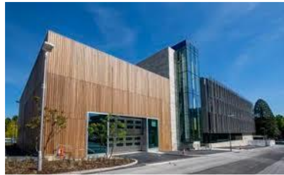
Fig. 5: New Lab Building, Chilworth Science Park
